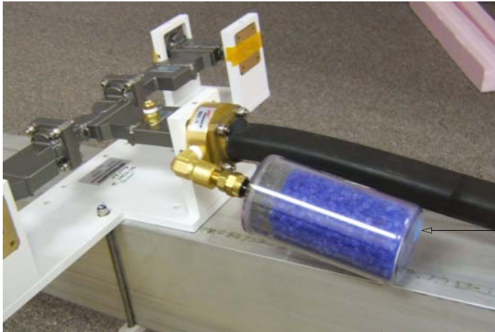
Figure 2-7 Install the desiccator cartridge (example for a 4" x 4" feed support arm)
