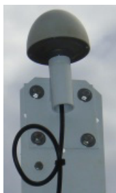
Figure 2-5 Mount the GPS antenna (shows optional bullet antenna)
