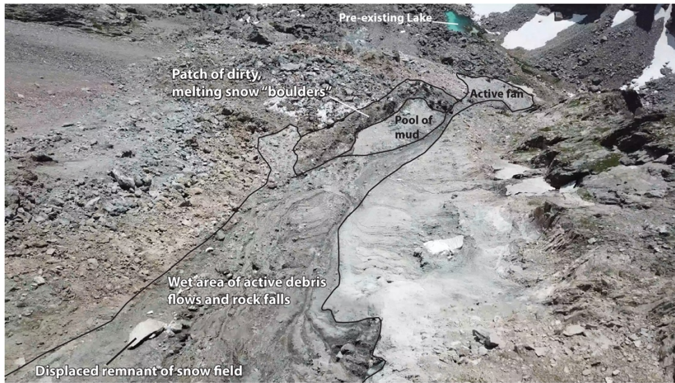
Fig. S10 Photo taken by the UAV on 15 July 2022 looking down the landslide from near the headscarp, showing the debris flows flowing into a pool impounded behind a dam of debris and snow 'boulders,' with some flows going around the right side onto the lower active debris flow fan.
