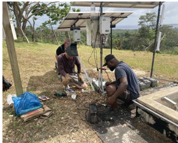
Reinstallation of the SANVU station (Vanuatu) in October 2023. Installation of the new T360 sensor in the cave (left) and integration of a new solar panel power supply (right).
