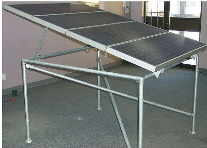
Figure 1 Completed assembly of a single bay support frame
