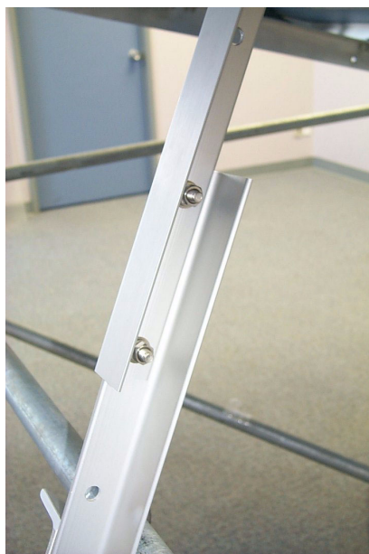
Figure 6 Attach the secondary support legs
